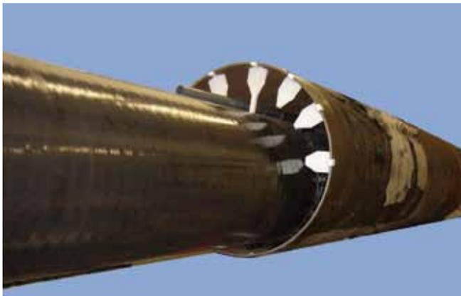
Fix plastic holders with clip on the inner wall of the casing pipe. Cut to suitable length if necessary. The distance must be chosen according to the recesses of the support segments.
