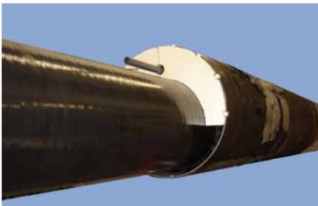
The cable duct has to be pulled through between the semi-circular recesses. If the recesses are too small, they can be slightly enlarged by cutting them out further with a knife.
