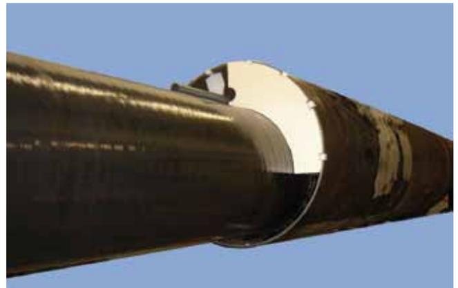
Place foam segments on the carrier pipe and insert into casing pipe. Hereby the raised flange rests on the outer front of the casing pipe. This means that secure support is guaranteed.
