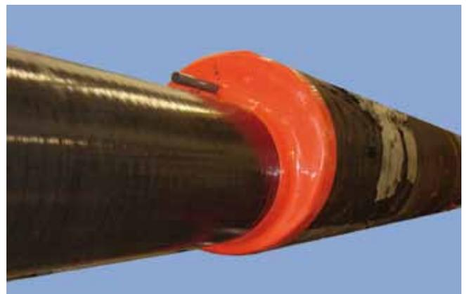
Pull casing end seal over the pipe and fit fastening straps (included).
