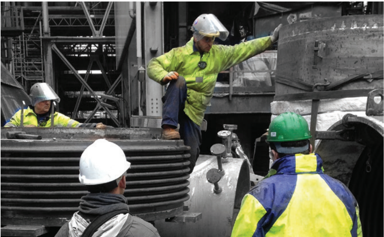
Supervising installation of FCCU Expansion Joints in a refinery in Spain
